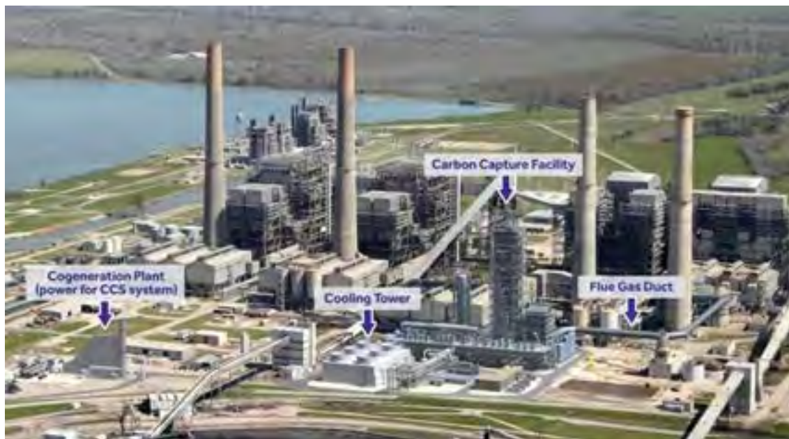
Figure 14-7: Layout of the CO 2 capture installation at the Petra Nova coal-fired power station in Texas (USA) (Source: U.S. Energy Information Administration)
